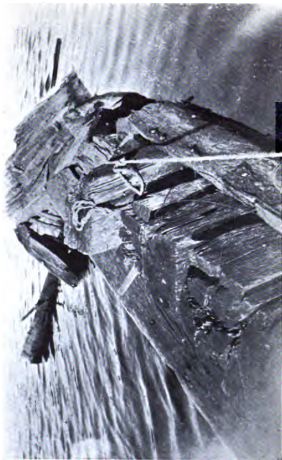
STEM AND FOREFOOT OF THE TWENTY-TWO GUN BRIG "JEFFERSON." One of the forty-day marvels of the speedy builder Henry Eckford. She was launched April 2, 1814, and is now sunk in Sackett's Harbour, opposite Shiphouse Point.
